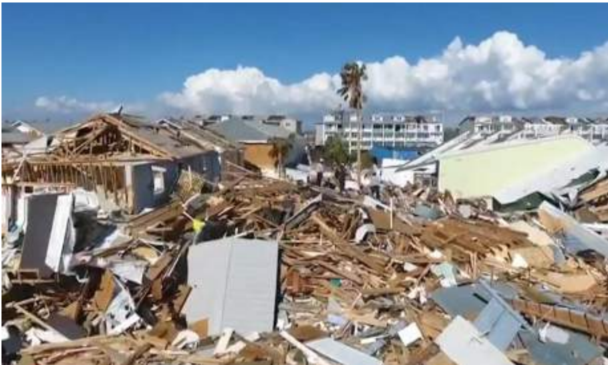
Fig. 8.2 Hurricane Michael damage. (Courtesy of Wikimedia Commons)
